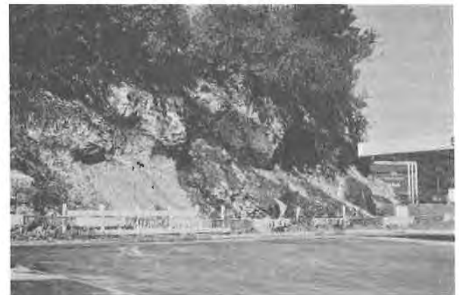
Figure 13. Oversteepened slope where limestone overlies weak shale (a. before failure; b. after failure).
