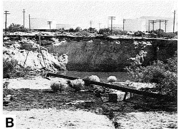
Figure 2. Local setting of the Wink Sink. (A) South side of the Wink Sink, June 5, 1980; view is to southeast from the northwest side of the hole. Area to the right (west) of brine pipeline (arrow) has subsided about 10 ft (3 m), producing a noticeable sag. (B) Wink sinkhole, June 5, 1980; view is to east from the southwest side of the hole. Pipeline in foreground was not in use when sinkhole formed. Oil pipeline on far side of sink was in use and had to be rerouted after being broken. Oil storage tanks in background are operated by Shell Oil Company.
