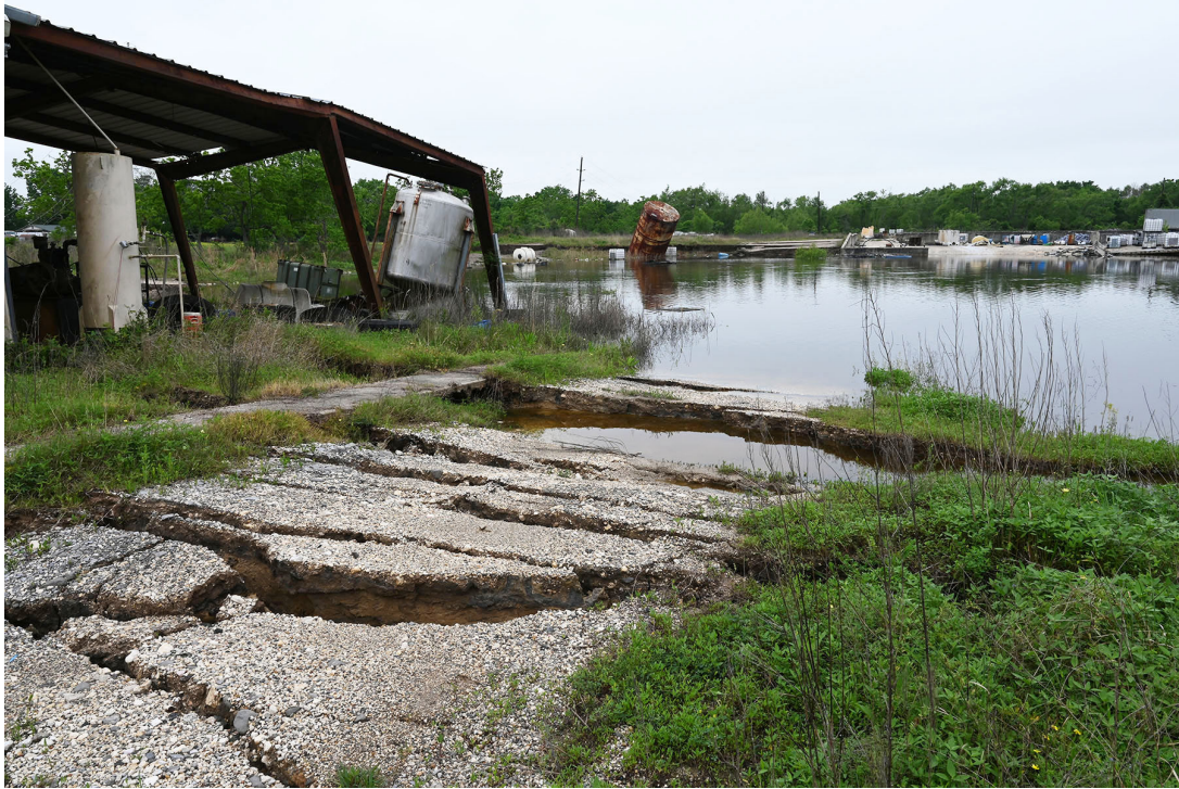
Figure 12. Fissures, scarps, and slump blocks on the east side of the April 2023 collapse area. View to the west across the 2023 sinkhole.
