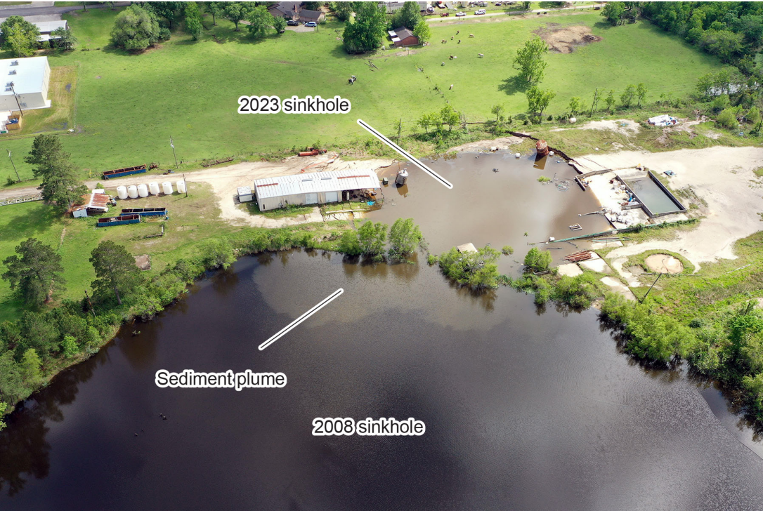
Figure 13. Oblique drone view to the south showing a sediment-laden plume of water flowing from the 2023 sinkhole into the 2008 sinkhole.
