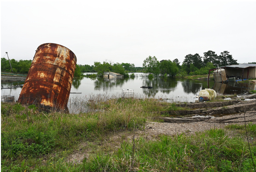
Figure 3. View to the northeast across the 2023 Daisetta sinkhole. The 2008 sinkhole is in the background beyond the tilted yellow-gray building.
