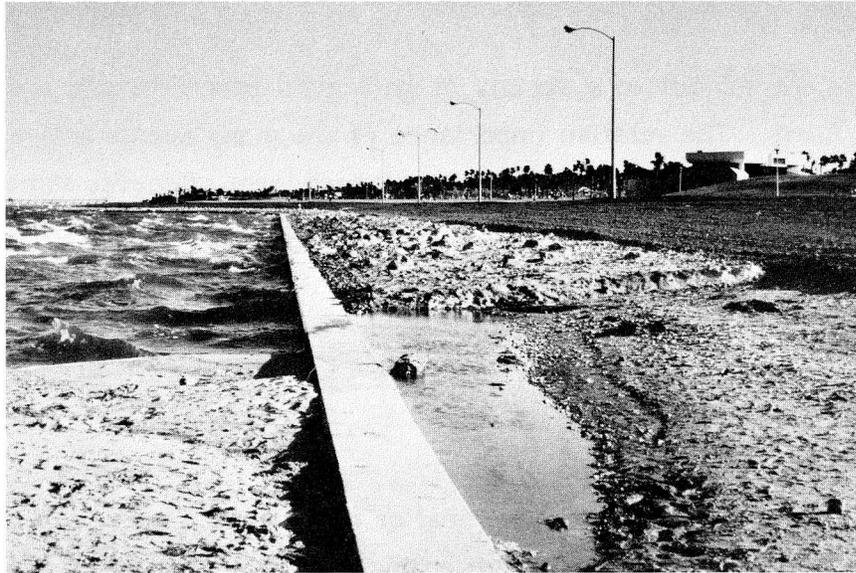
Figure 11. Low concrete bulkheads backed by consolidated riprap and graded fill at Cole Park, southern Corpus Christi Bay.
