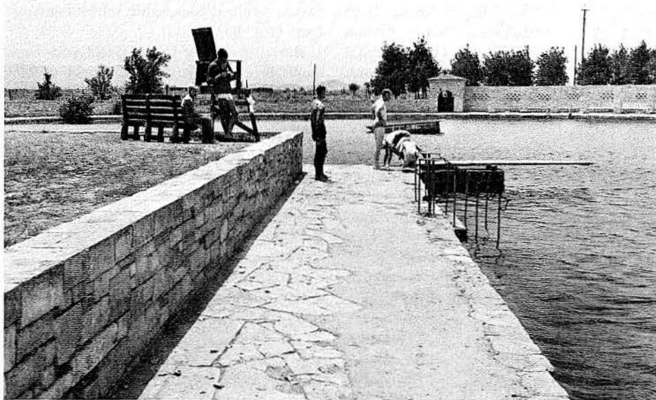
FIG. 25. The Balmorhea swimming pool which incorporates the total flow of San Solomon Spring. The spring was used by the Indians and frontiersmen and later for irrigation. Prior to the building of the masonry walls and walks of native Boquillas Flagstone, the water issued from a large swamp. (Photograph by Texas Parks and Wildlife Department.)
