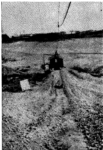
FIG. 5. CLAY EXCAVATION BY DRAG-LINE METHOD AT BRICK PLANT AT FERRIS, TEXAS
