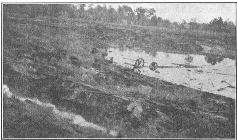
Fig. 3. View taken October 28 looking northeastward. Note boiler at water's edge. In photograph of October 9 (Fig. 2) this boiler is seen on undisturbed land, the bank having in the meantime slumped and the earth moved sinkwards. The power house seen in the previous photograph has been removed, the foundation having been disturbed by slumping. (Photograph by Fenn.)
