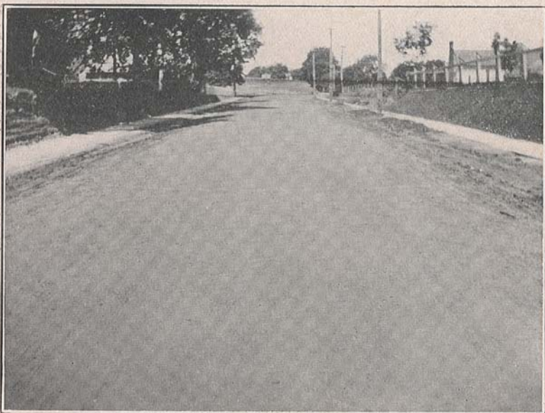
Plate 18. Iron Gravel Road at Henderson, Rusk County. Built with Gravel No. 2654.
