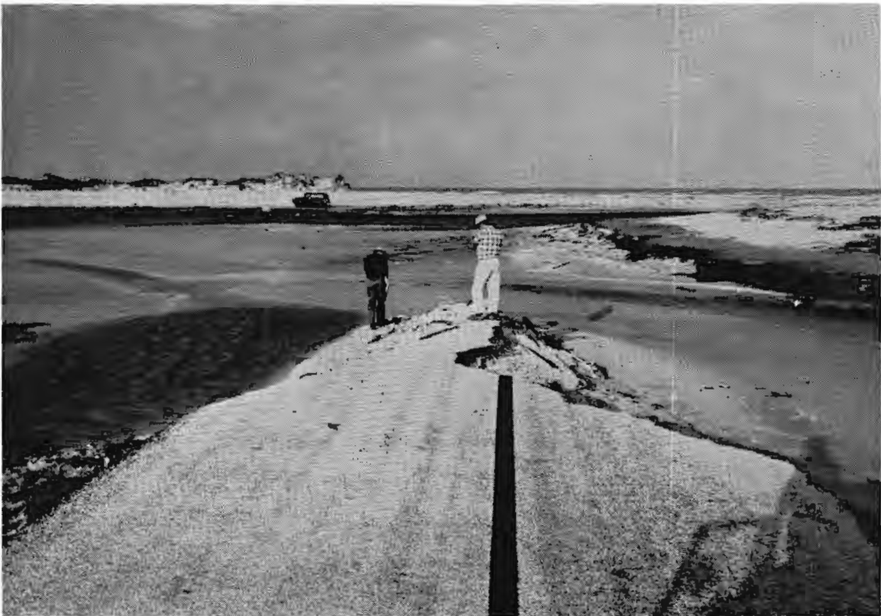
Geologic forces in action. Hurricane Carla struck the Texas Coast in September and provided dramatic evidence of how natural forces shape the land. The photo shows a new channel cut through a paved road on Mustang Island.
